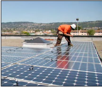
Installation of solar photovoltaic panels
