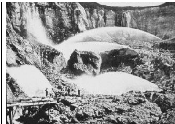
Figure 3. As part of hydraulic mining, monitors (i.e., water cannons) were used to break down the gold-bearing gravel deposits. The monitors were so powerful, one observer explained, that they would "toss about rocks, tons in weight, as if they were mere pebbles."
